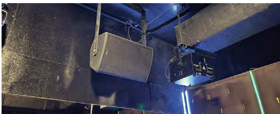
Wall-mounted NEXO P15s cover the outer areas
